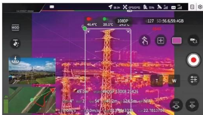
Support point temperature measurement, area temperature measurement and high temperature alarm
