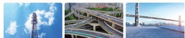
Communication Facility Inspection
